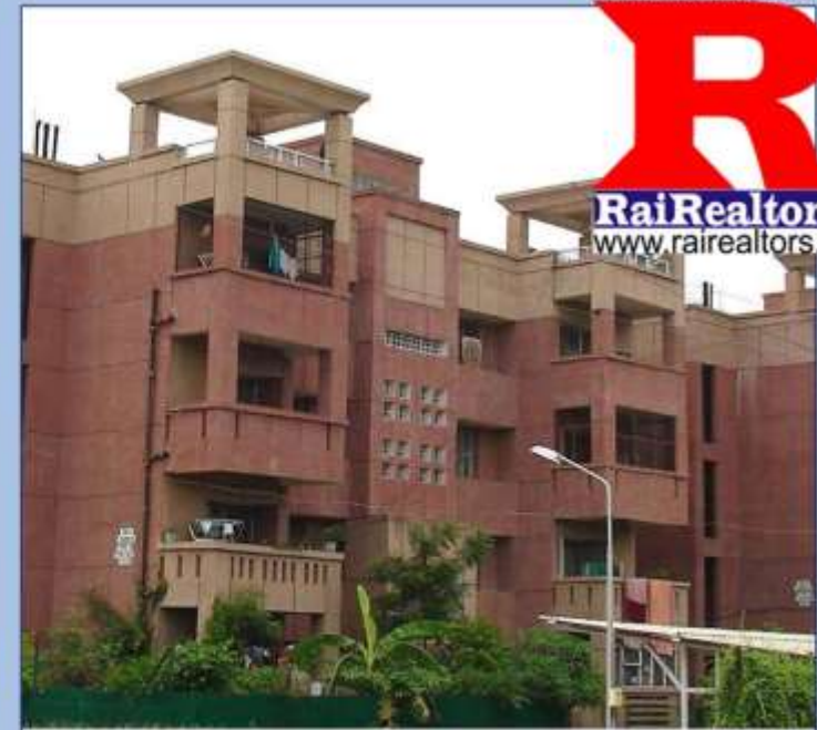
200 Residential Apartments, AIIMS, Ayurvigyan Nagar
