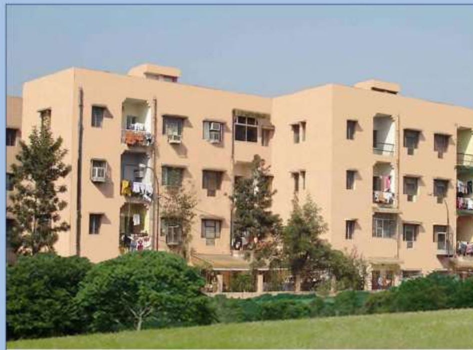
770 Apartments, Sector-18, Rohini, Delhi
