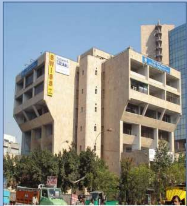
Office Building, Laxmi Nagar
